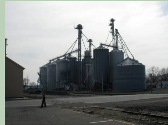
Grain elevator in Bargersville
