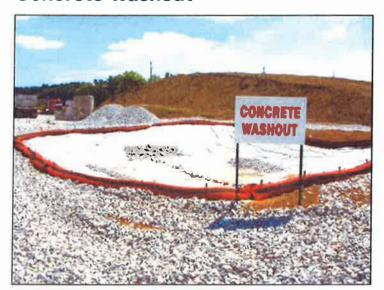
Concrete washout areas are designated locations within a construction site that are either a prefabricated unit or a designed measure that is constructed to contain concrete washout. Concrete washout systems are typically used to contain washout water when chutes and hoppers are rinsed following delivery.
