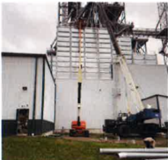
Original Photo of Site Shown Below
