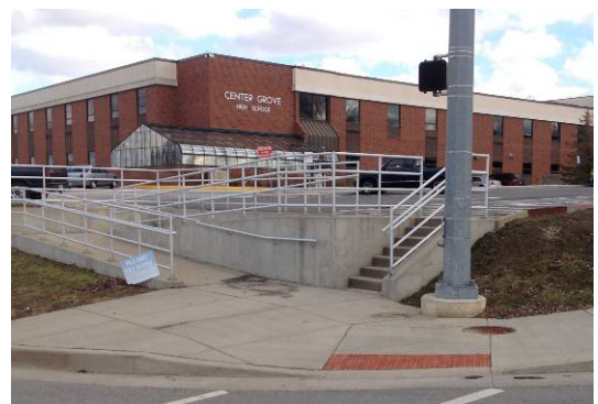
Example of utility pole obstructing ramp landing
