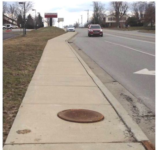
Example of displacement at utility
