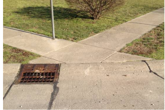
Example of poorly located drainage structure, lack of ramp, and a non-compliant grate
