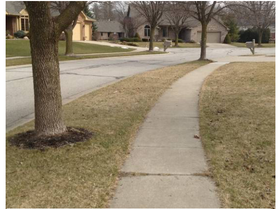
Example of displacement of sidewalk at tree
