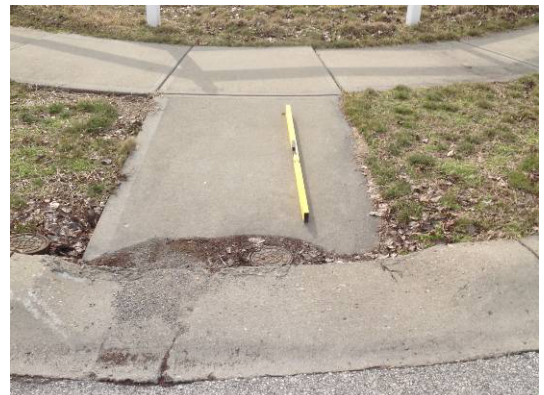
Example of settlement at curb and utility along with degradation of pavement
