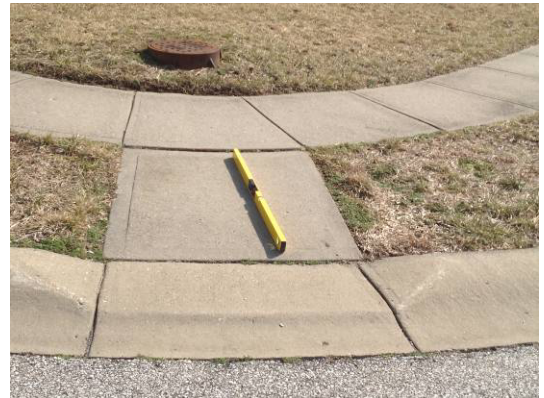
Example of +\frac{1}{2} " displacement at gutter line and horizontal displacement at top of ramp
