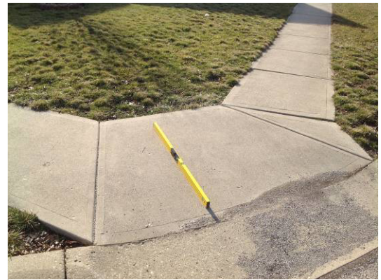
Example of lack of turning space and landing
